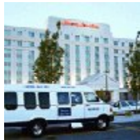
Hampton Inn and Suites/ Chicago North Shore 5201 Old Orchard Road Skokie, Illinois 60077 Phone: (800) HAMPTON
